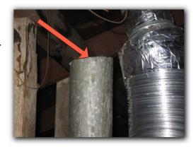
Iron drain pipe in crawl space for toilet has corrosion, which can be insignificant surface corrosion, have limited life expectancy, or be in need of replacement. Although insignificant surface corrosion is common, some corrosion may be at risk of causing leaks when iron pipes are this old. If the more comprehensive evaluation that can be provided by a plumbing contractor is desired, contact a qualified, state licensed plumbing contractor.
