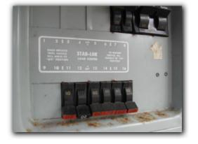
Circuit breaker labeling for main panel is incomplete. Labeling which appliance/circuit each breaker controls allows shut-off of the intended circuit, which can avoid shock/electrocution when working on wires that are assumed to be shut off. Recommend that this finding and all associated components be reviewed, and corrected as needed, by a qualified, state licensed electrical contractor.
