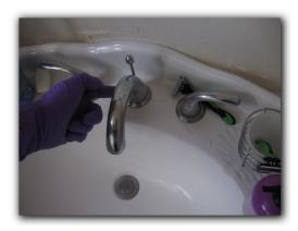
Handles for sink faucet in rear bathroom are difficult to operate. Recommend that this finding and all associated components be reviewed, and corrected as needed, by a qualified, state licensed plumbing contractor.
