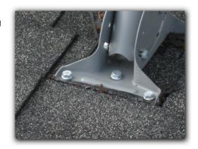
Metal has been installed on roof. Possible previous hatch noted in attic below. May increase risk of moisture intrusion. Recommend seller disclose any known history, including any evaluation/repair documentation or permits, in order to assist buyer in determining current condition and confirm proper repairs, which may require review by an appropriate, qualified, state licensed contractor/specialist.
