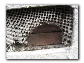
Opening at left rear corner of building has separated screen, possibly allowing pest intrusion, such as rodents, which can cause damage and increase health risk. Recommend that this finding and all associated components be reviewed, and corrected as needed, by an appropriate, qualified contractor.
