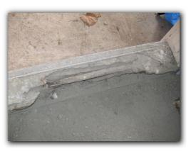
Front wall has apparent water intrusion at floor, which may cause deterioration of building materials within or promote microbial growth. Recommend that this finding and all associated components/areas be reviewed, and corrected as needed, by a qualified, state licensed General contractor or other appropriate, qualified contractor.
