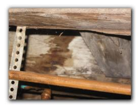
Wood ("cellulose") debris noted in crawl space at a number of locations. Wood can attract wood boring insects to building wood framing, which can cause damage and compromise the structural integrity. Recommend removal of any scrap wood in crawl space by a qualified person.
