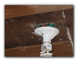
Junction box at left rear corner of building adjacent to garage has cover plate missing, exposing current-carrying components and creating a risk of shock, electrocution, or spreading any junction box fire. Recommend that this finding and all associated components be reviewed and corrected as needed by a qualified licensed electrical contractor.
