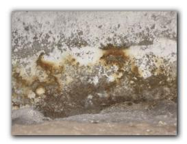
Corroding rebar can expand and damage foundation. Exterior grade does not slope away from building. Recommend that the foundation be reviewed, and monitored on a regular basis, by a qualified, state licensed foundation contractor. Recommend reducing water exposure by improving drainage on grounds. Recommend using appropriate, qualified, licensed contractors.
