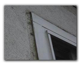
Opening on right wall near kitchen may allow moisture intrusion, which may cause deterioration of building materials within wall and promote microbial growth. Recommend that this finding and all associated components/areas be reviewed, and corrected as needed, by a qualified, state licensed General contractor or other appropriate, qualified contractor.
