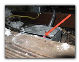
Low voltage wiring extends over attic entrance, causing wiring to be at risk of damage & disconnection and creating risk of injury to persons during opening/closing attic door or when entering/exiting attic. Recommend having wiring moved by the relevant company.
